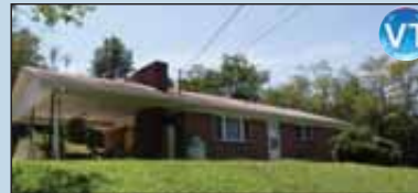
LEICESTER! All brick home w/3 BR, full bsmt, carport, large living room w/FP central air, views, garden space, minutes to downtown Asheville, MLS#492696, Code#3572, $180,000!
